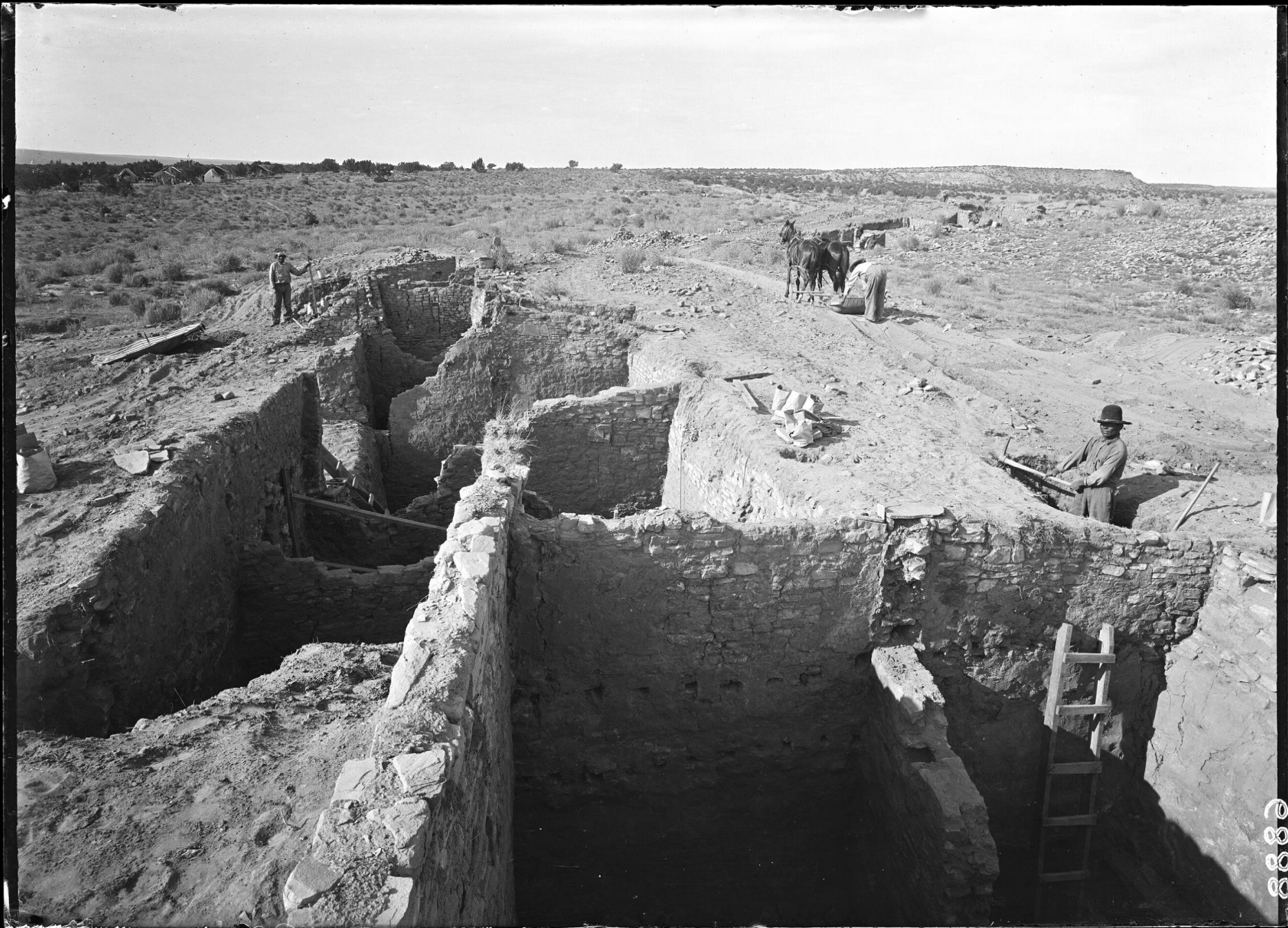
Excavation of Hawikku's ruined houses in 1920.
