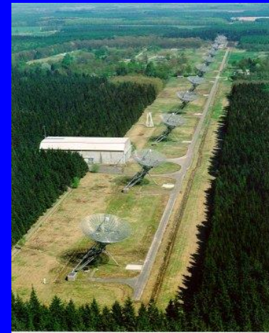
Upgraded WSRT in The Netherlands
